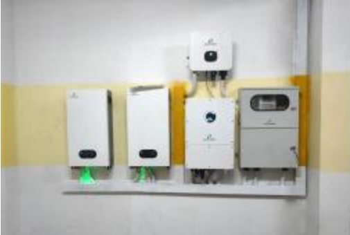
C&L 10KW / 20KWh The energy storage system is located in the Gambia.
